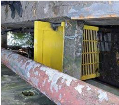
Installation of filters in water drainage
